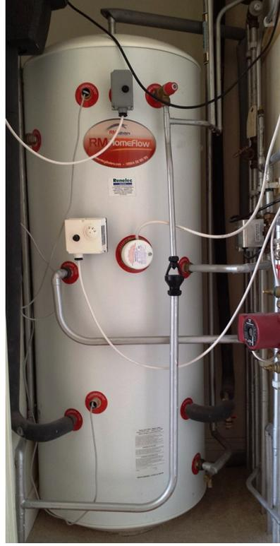
Figure 2.7: Heat storage tank in a smart solar tank system connected to solar thermal collector on building roof.
