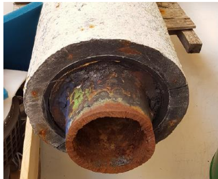
Subsea Oil Pipe
